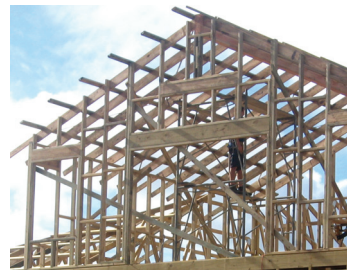
A Building under Construction
