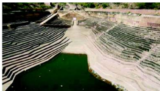
Fig. : A Traditional Method of Rainwater Harvesting
